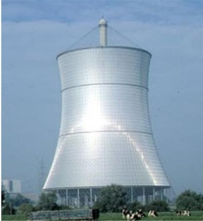
Figure 1: A similar cooling tower in Germany, but with vertical and horizontal instead of inclined cables.
