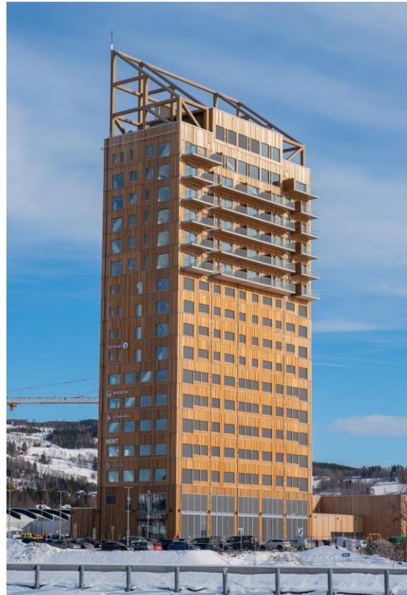
Figure 1 - This building is made entirely from wood.
